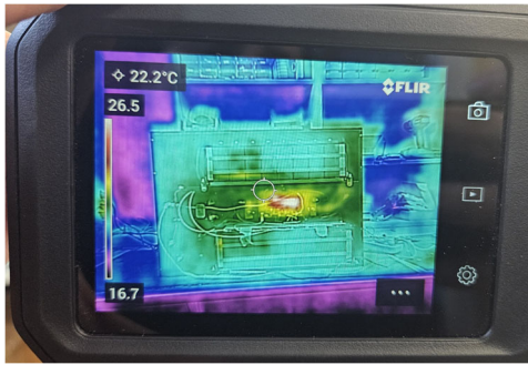
Fig. 17. Thermal camera results under low load
